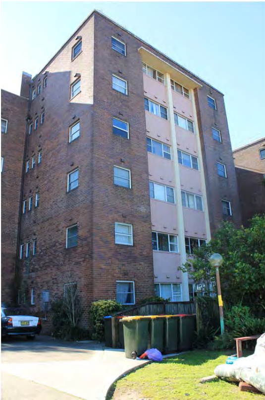
Figure 5 Six (6) storey residential flat building to the immediate east of the site
